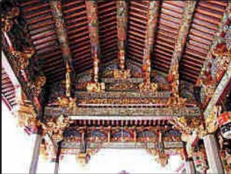
The main truss of the Prayer Pavilion
