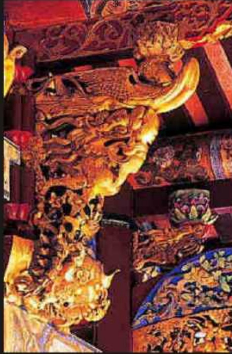
The Cantilevered Base and Bracket
