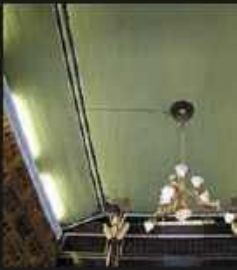
The trapezium ceiling in the Soo and the Ee Kok Tong is not typical of the Southern architecture
